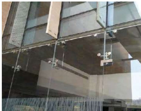
Ambience Tower, Gurgaon
